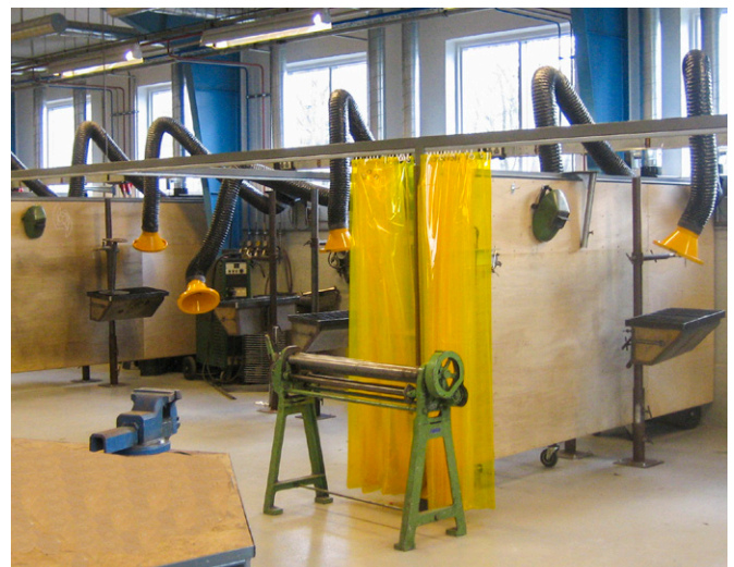
Wing arms ø160mm 3m installed at technical school. Including automatic control devices for automatic start/stop of fan and motor damper.
