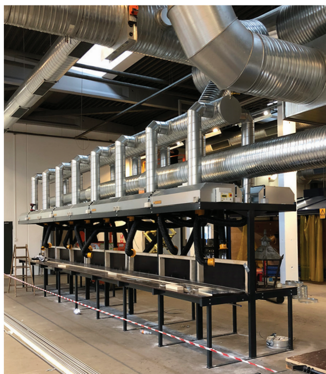
As seen in the picture, the hoods can be mounted in series so that the length of the hood itself can almost become infinite.
