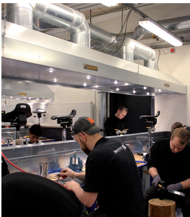
Extraction Hood at a school
