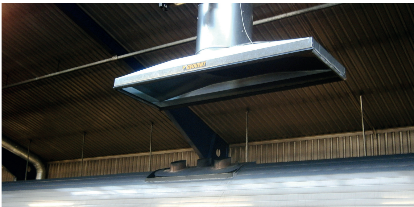
Extraction Hood for train
